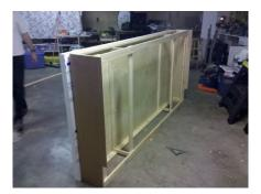
The first thing we built was a frame out of 1x3's and skinned the front and sides for the bottom section of the fireplace. We made the front two 1x3's flat and the back two 1x3's on edge; we did this so if the fire box is put in place, the 1x3 wouldn't be in the way.
